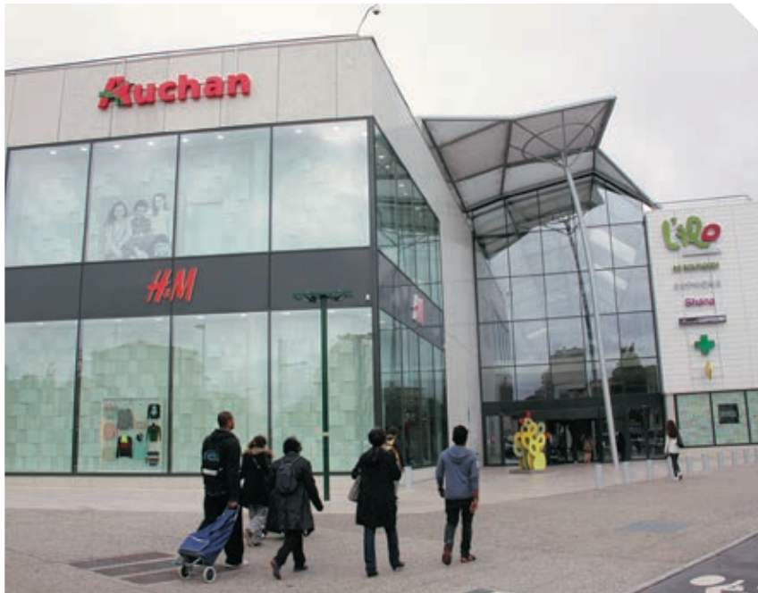
Centre commercial L'Ilo
